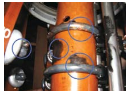
Fig. 3: Blue phase tapping leads and broken cleats.
