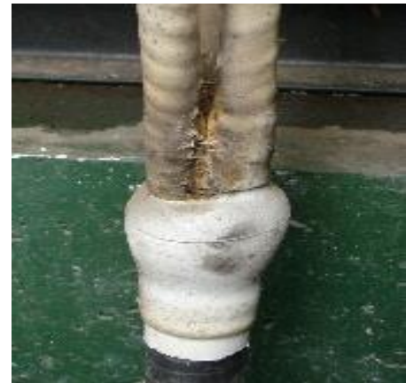
Figure 10: Inspection on cable terminations
