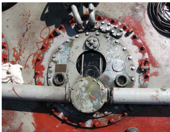
Figure 1: Pressure relief plate blown out from B phase diverter head cover
