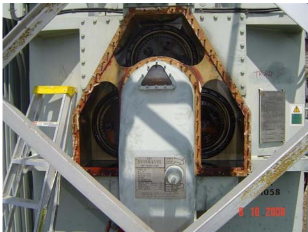
Figure 18: View of the Ferranti DS2 tap changer with cover removed
