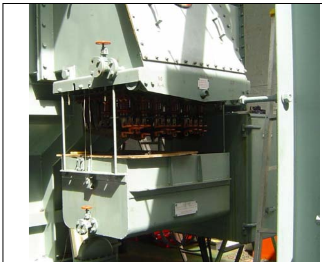
Figure 24: Diverter shown opened below and
