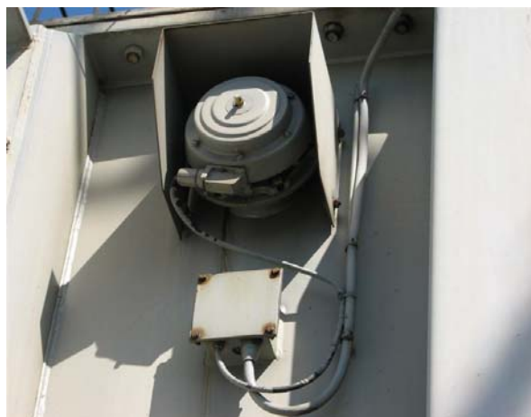
Figure 2: Main tank pressure relief valve operated (yellow pin sticking out)
