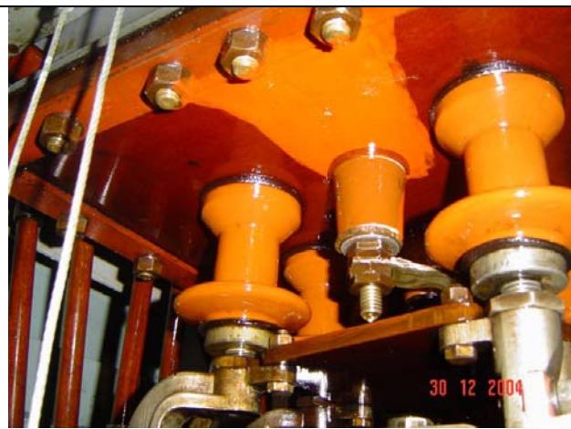
Figure 23: Barrier board and insulator after repairs
